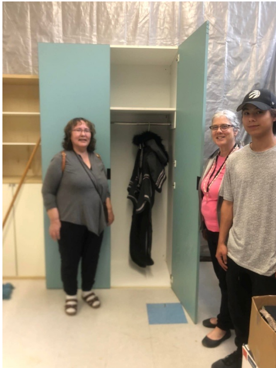
Installing a closet for sewing samples
